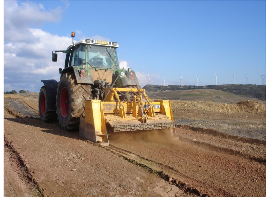
Mixing of steel shots
