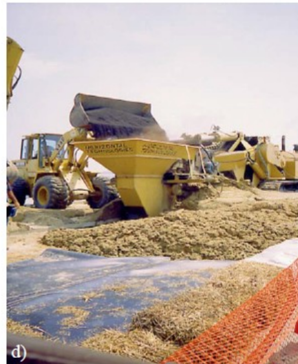
Figure 4-1. Examples of ZVI and ZVI emplacement: (a) fine-grained ZVI, (b) coarse-grained ZVI being placed in a trenched PRB, (c) microscale ZVI in an injectable EHC ® slurry, and (d) installation of ZVI PRB at a U.S. Coast Guard facility using a one-pass trencher.
