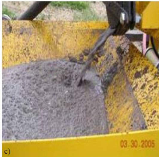
Figure 4-1. Examples of ZVI and ZVI emplacement: (a) fine-grained ZVI, (b) coarse-grained ZVI being placed in a trenched PRB, (c) microscale ZVI in an injectable EHC ® slurry, and (d) installation of ZVI PRB at a U.S. Coast Guard facility using a one-pass trencher.
