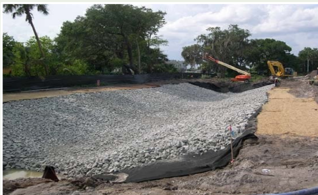
Recycled concrete for erosion control
