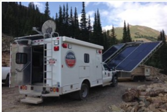
A mobile solar system to power tools
